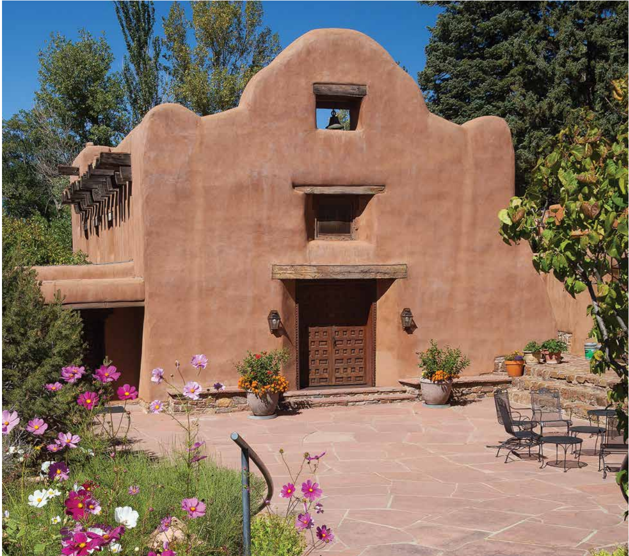
SAR's administration building was originally the home of Amelia Elizabeth and Martha Root White. The sisters commissioned architect William Penhallow Henderson to model their home after the church at Laguna Pueblo.
